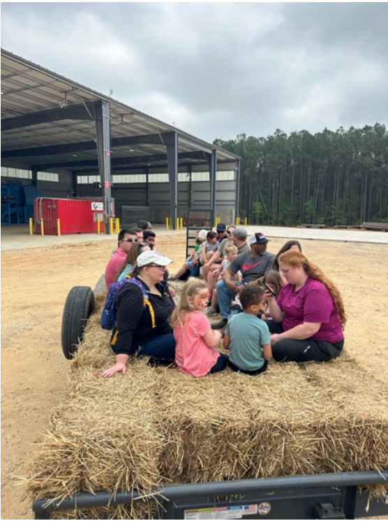
Photo Image 1: Hayride tour of the under construction MRF.
